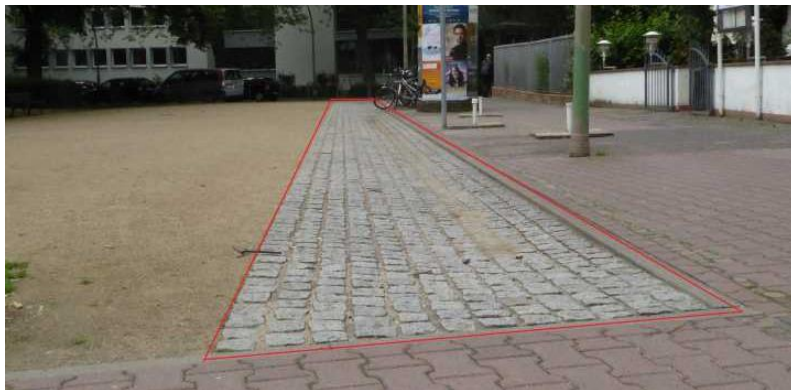
It is easier when the stones are arranged rectangular.
